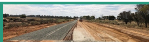
Stabilisation work on Dowerin-Kalannie Road
