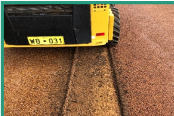
Finished edge for shoulder grading
