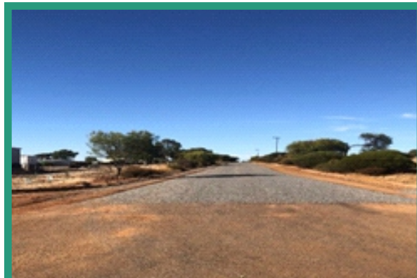
Central Road Prime and 14mm seal was laid in March
