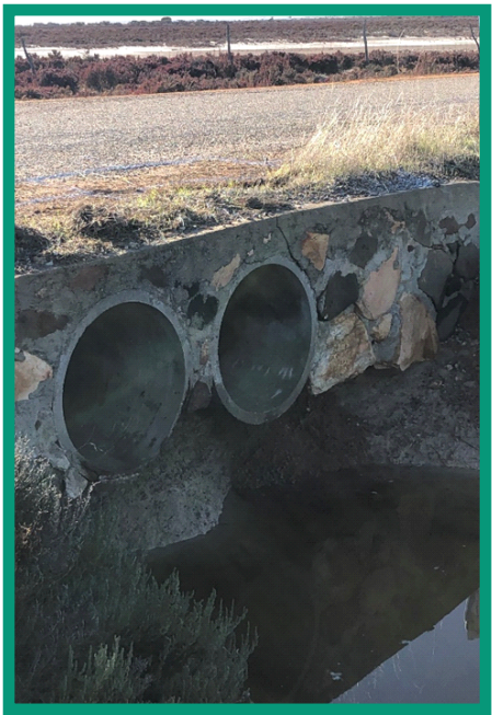
Washed out headwall, Kondut South East Road and reparation work.
