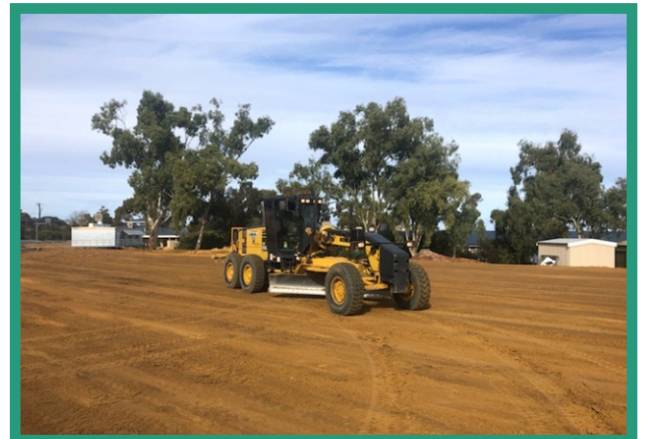
School hockey oval being graded and levelled
