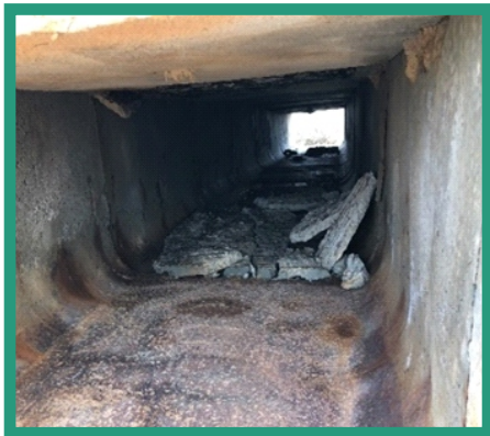
Newton Road box culvert sections in complete disrepair
