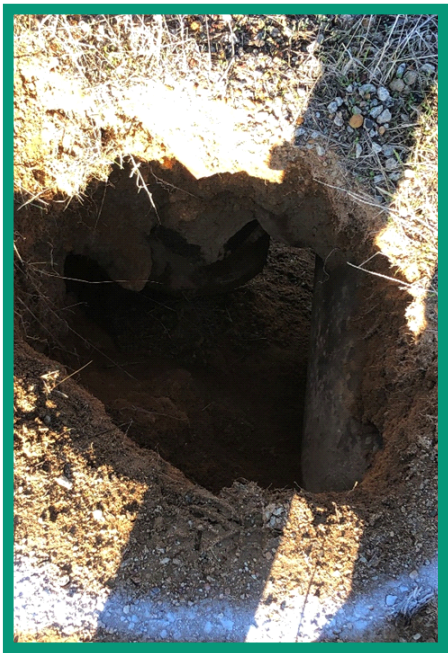
Washed out headwall, Kondut South East Road and reparation work.
