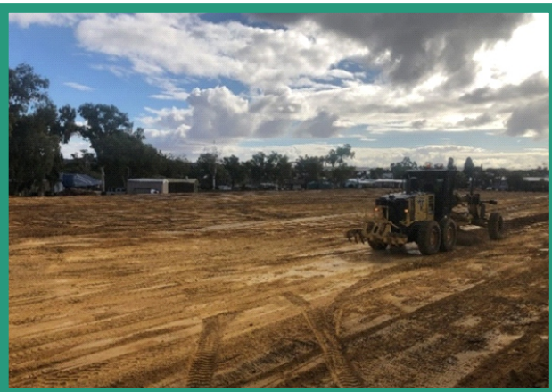
School hockey oval being graded and levelled
