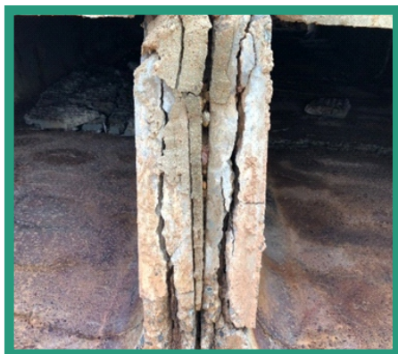
Newton Road box culvert sections in complete disrepair
