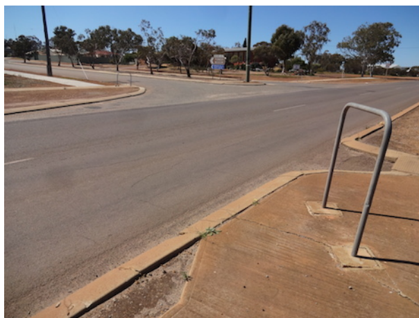
Kerb ramps, and short sections of new path, are required in some locations to ensure a smooth transition from path to road surface.
