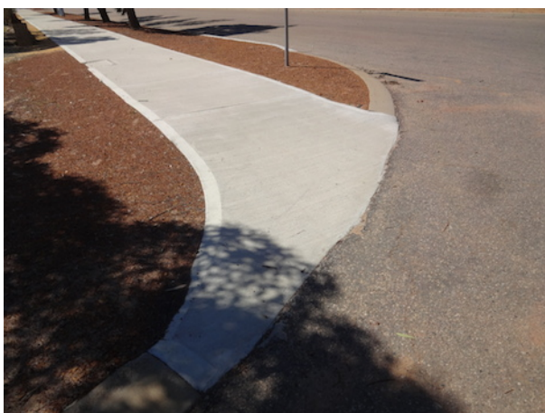
Smooth kerb ramps ensure a good transition from path to road for cyclists, gopher users, parents pushing prams and for those in wheelchairs.
