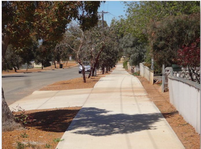
Most recently constructed paths in Wongan Hills are 2.0m wide, eminently suitable for the existing and future usage levels.
