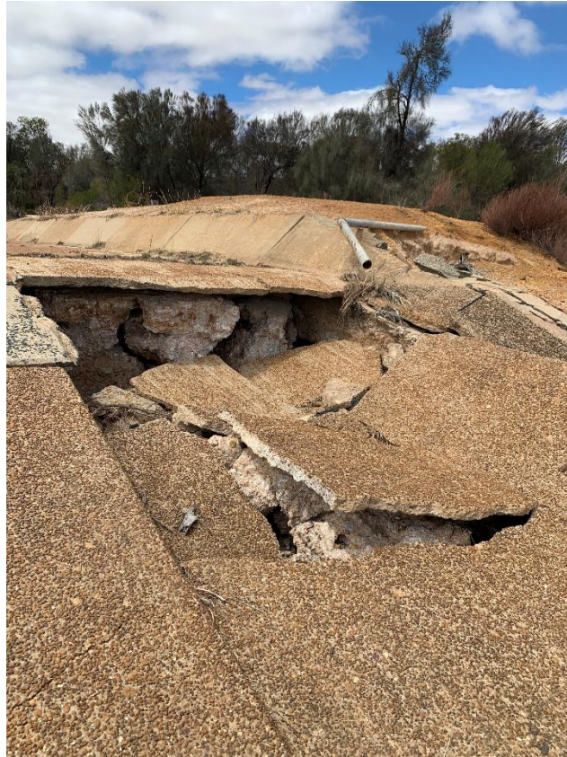
Damage to Existing Spillway
