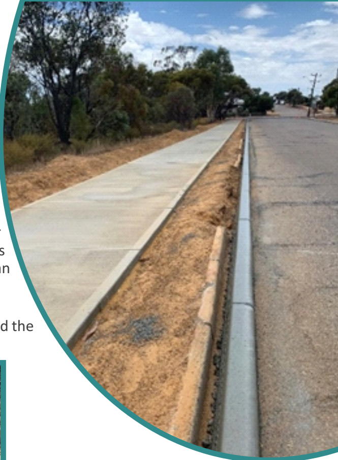
New kerbing and footpath Parker Place
