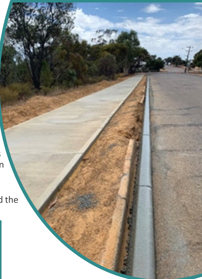
New kerbing and footpath Parker Place
